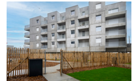
Orchestra (Doulon) 20 logements Barré-Lambot Architectes
